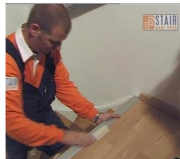
**Oops!** you need to have finished the flooring on the landing before you glue the stair head in place and the profile is designed to overlap the finished floor.
