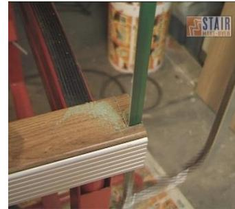
apply a bead of glue to both inside surfaces, mist the glue with water as you did with the treads, and press firmly into position at the top of the stairs. Use several strips of masking tape to hold the top stair profile in position whilst the glue dries
