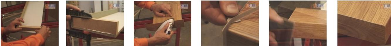
the tread is now ready to glue in place once all the treads and risers for the complete staircase have been cut to size and numbered as shown in the stair make-over laminate flooring for stairs general installation guide
