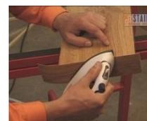
the risers are now ready to glue in place once all the treads and risers for the complete staircase have been cut to size and numbered as shown in the stair make-over laminate flooring for stairs general installation guide
