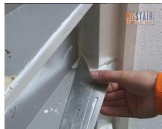
when you have the rough positions indicated by the arms of the measuring tool add the nut and tighten loosely before double checking the position of the arms and tightening securely to avoid the arms moving, the tool can also be used to measure straight treads if needed
