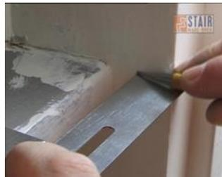
now take the centrepiece of the measuring tool and position over the nose tool towards the middle of the front of the tread and place measuring arms and large washer over the centre threaded stud to rest against the pencil marks at either side at the front, the back corners of the tread and any intermediate points (like a newel post).
