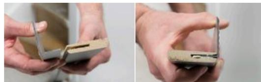
Apply glue into the groove of the new stair nosing and press the aluminium profile firmly into the groove
