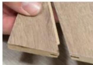
wipe off any excess glue immediately, and apply several strips of masking tape across the joint to prevent movement during drying once dry install as any other tread
